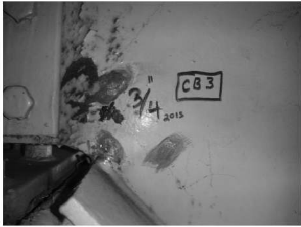
TYPICAL CB CRACK
