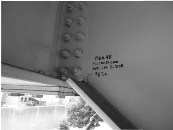
TYPICAL CB CRACK
