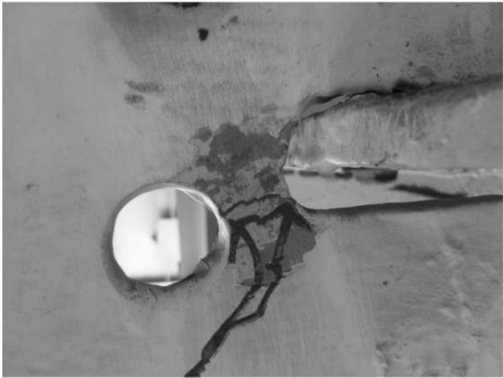
TYPICAL GP CRACK
