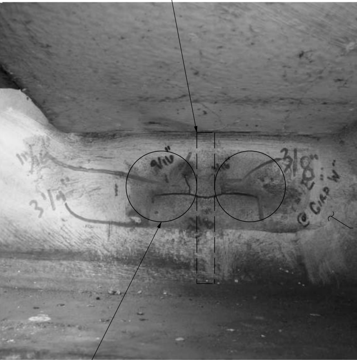
CX2 CRACK RETROFIT
