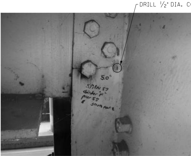
TYPICAL CC CRACK RETROFIT
