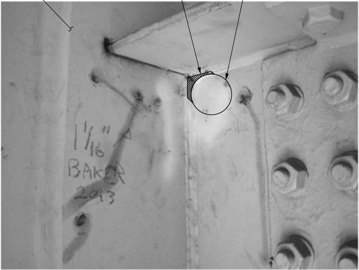
TYPICAL GF CRACK RETROFIT
